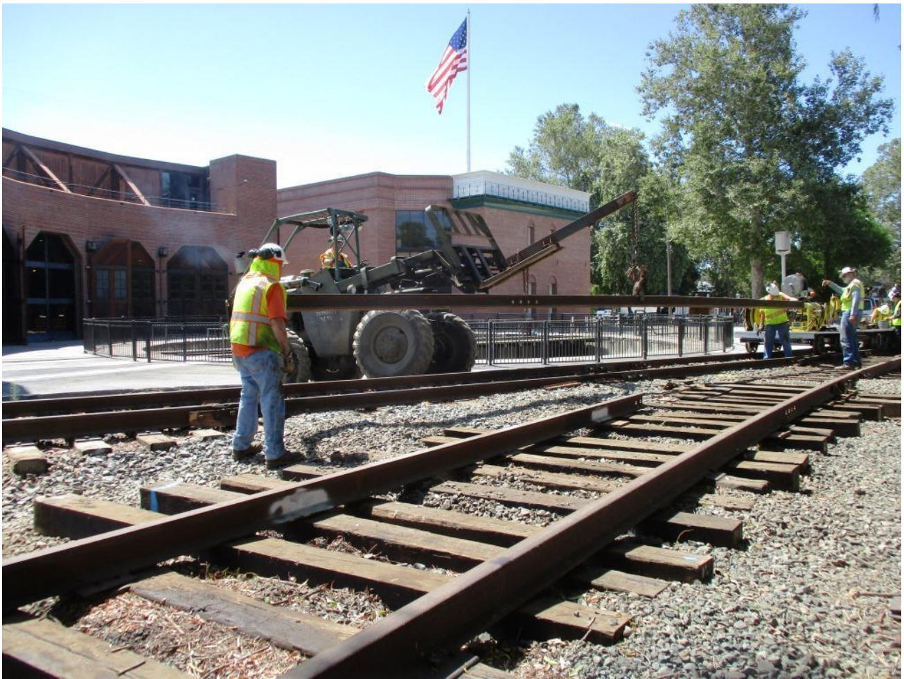
Alan directs the placement of the diverging stock-rail as Mike F. on Big Green brings it into position guided by Bill and Clem
