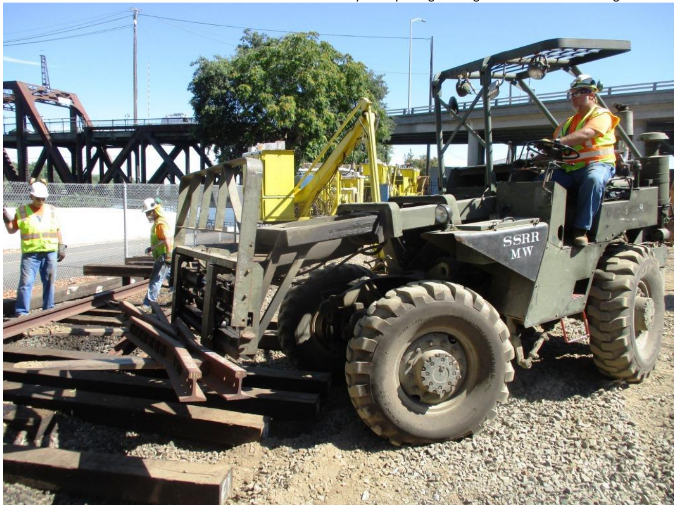
Speaking of the frog, with the rail cut and removed, Mike F. on Big Green brings it in
