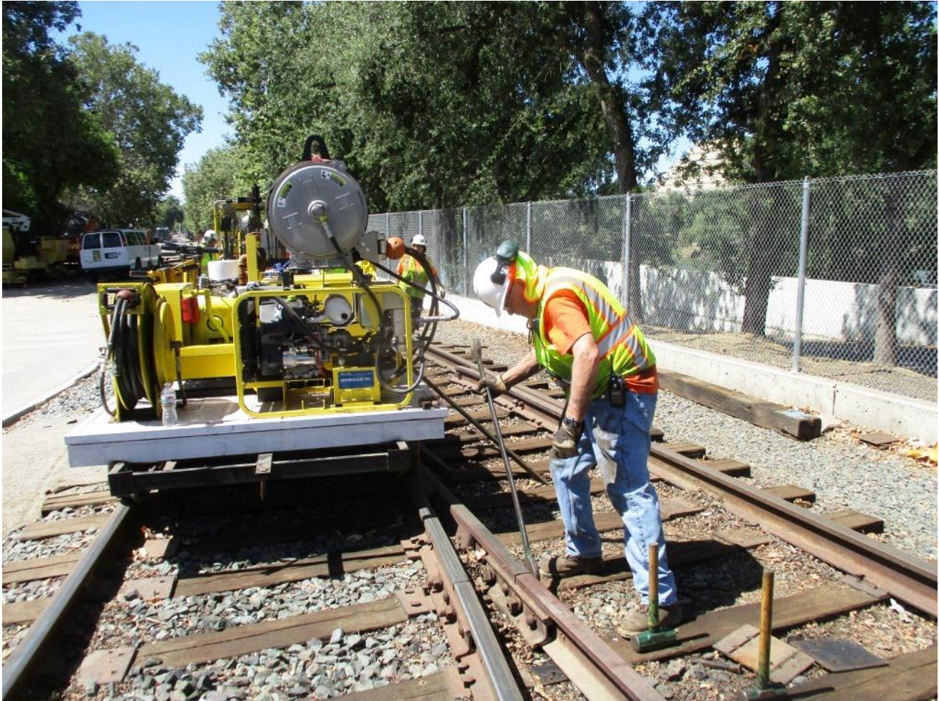
With the diverging stock-rail in place, Bill tightens the bolts
