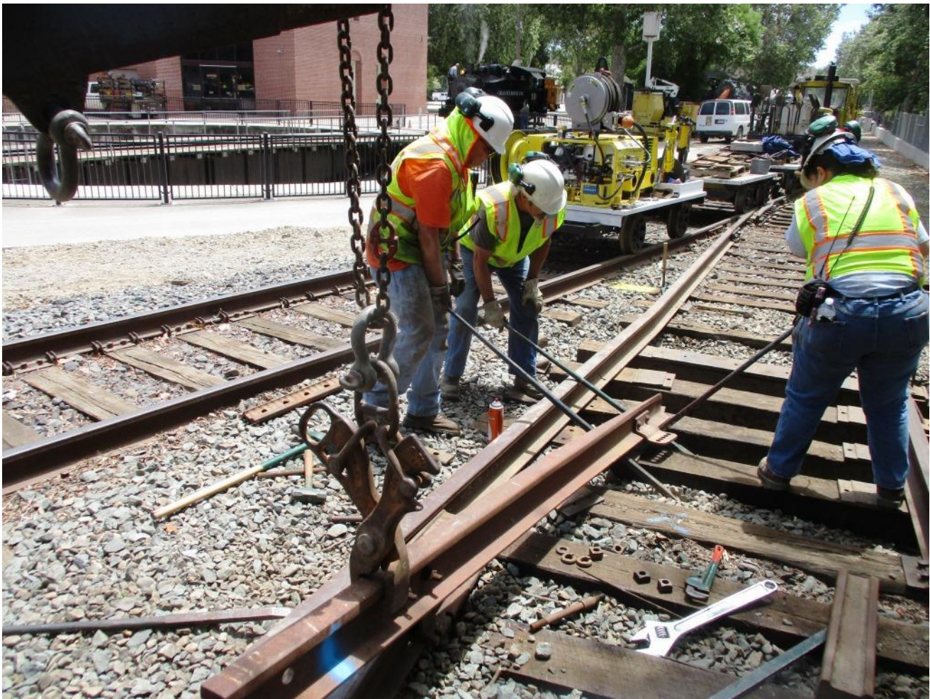
Bill, Ed, and Heather use lining bars to maneuver the switch-point
