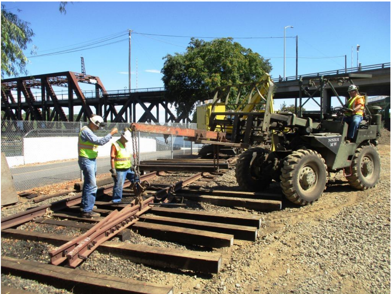
Alan guides Mike F. on Big Green with the "stinger" attachment for the precise placement of the frog
