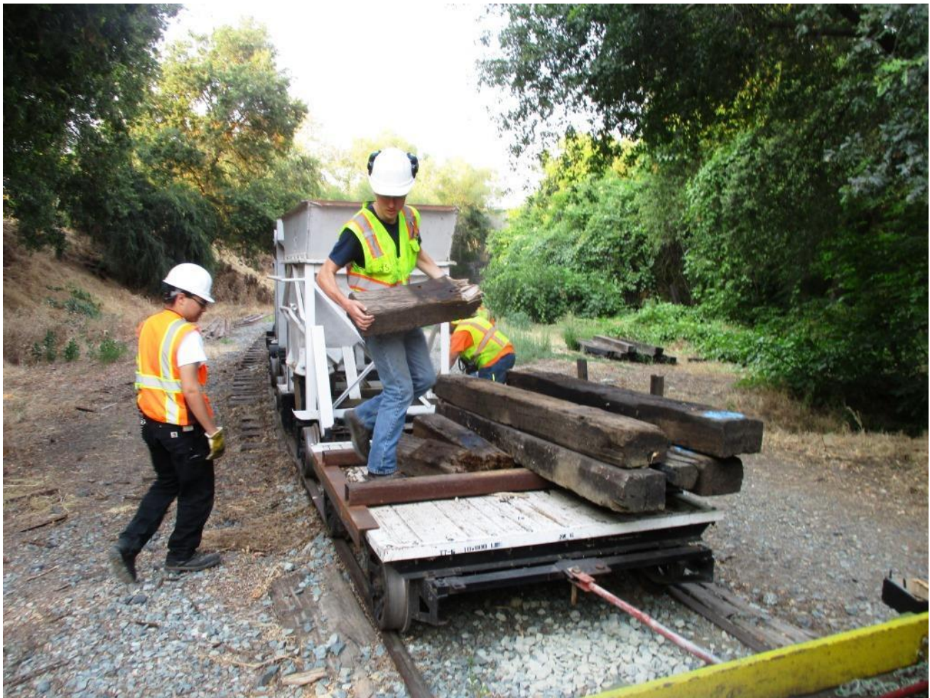
Jack starts the dead tie disposal with the broken bits
