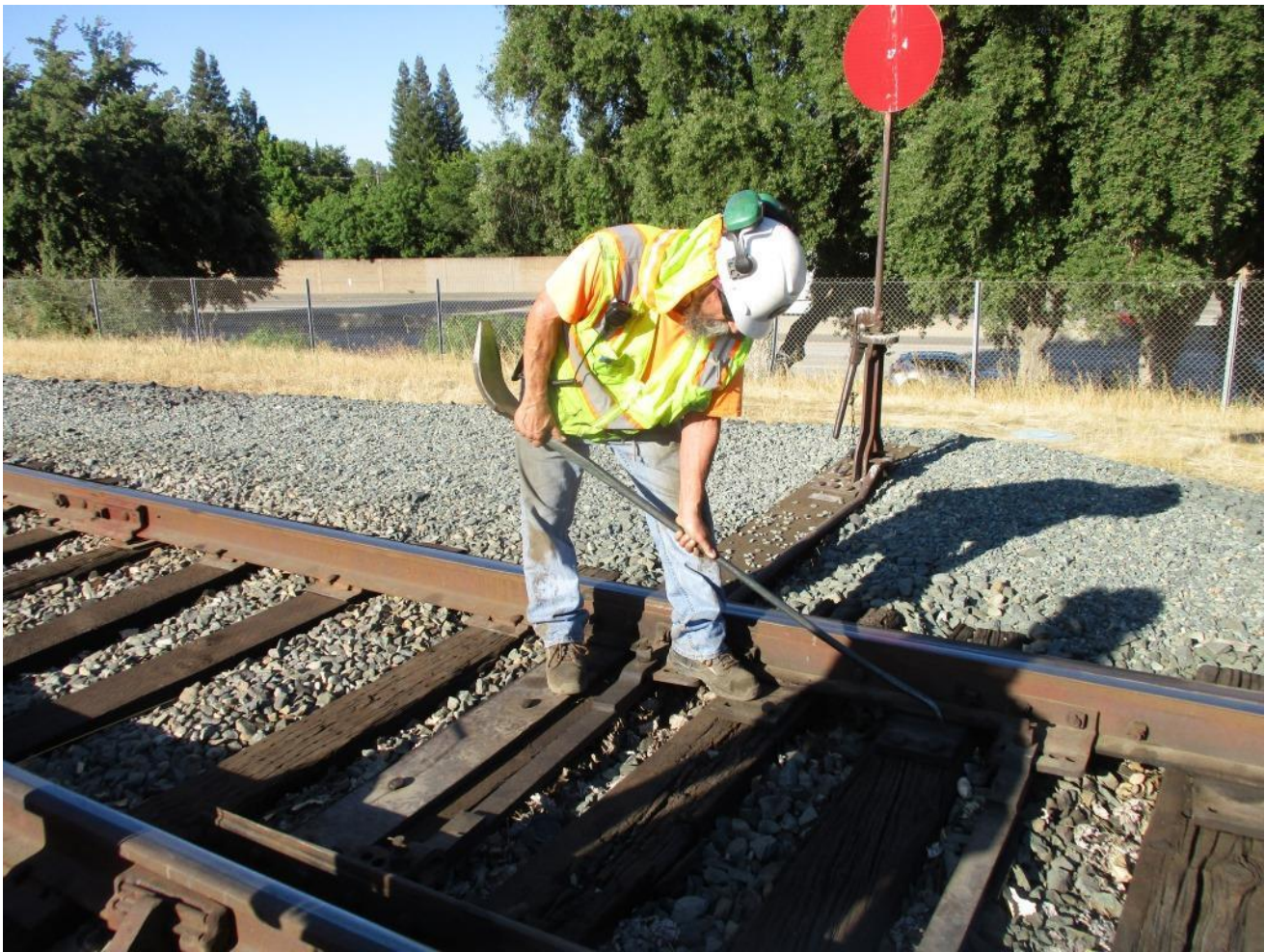
Joe scrapes debris off the switch plate at Switch 17
