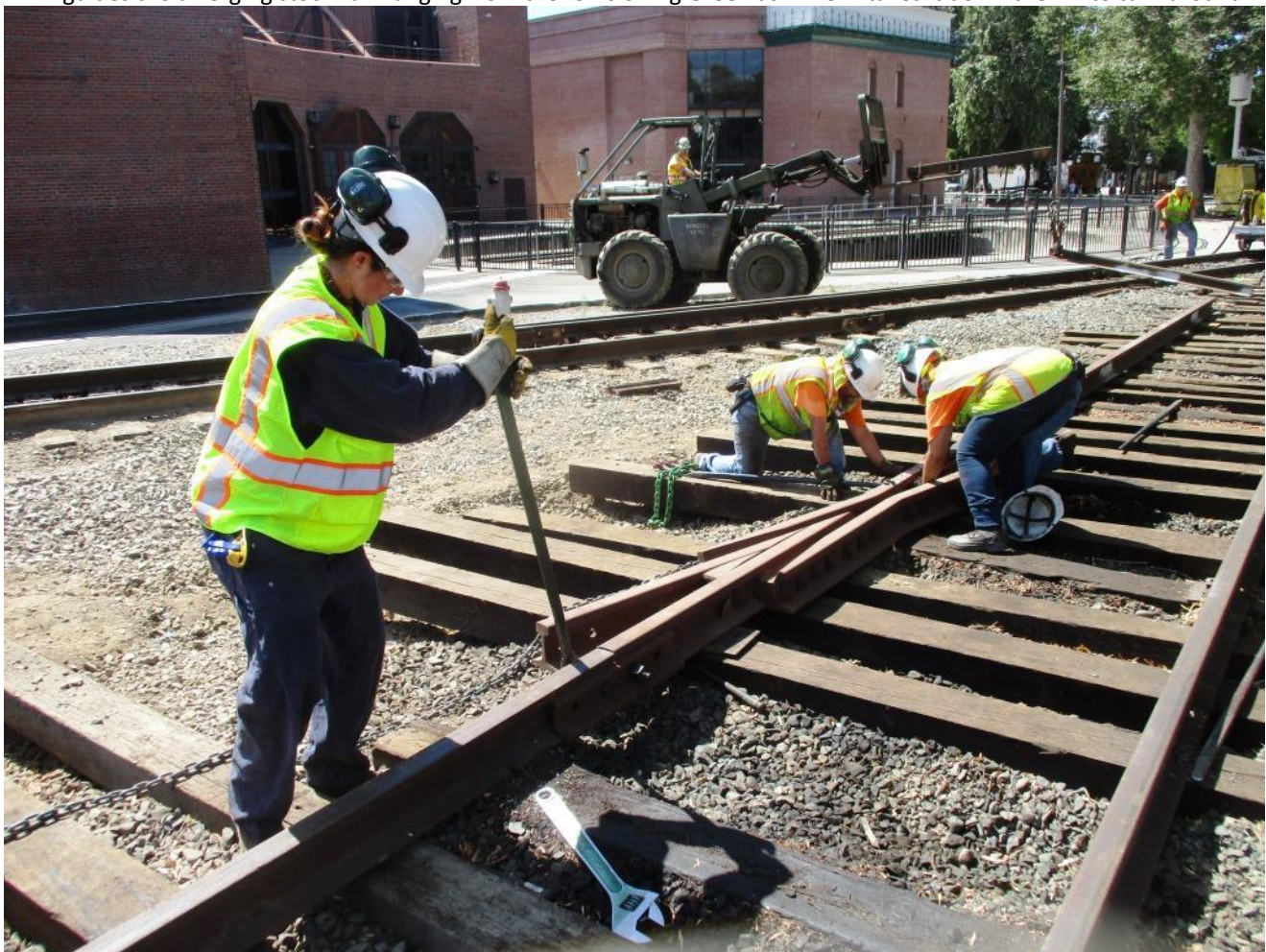
Samantha tightens bolts at the north end of the frog while Joe and Pam work on the south end
