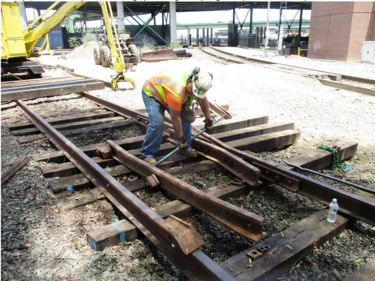
Meanwhile, back at the frog, Mike F. uses a lining-bar to shove the guard-rail into place
