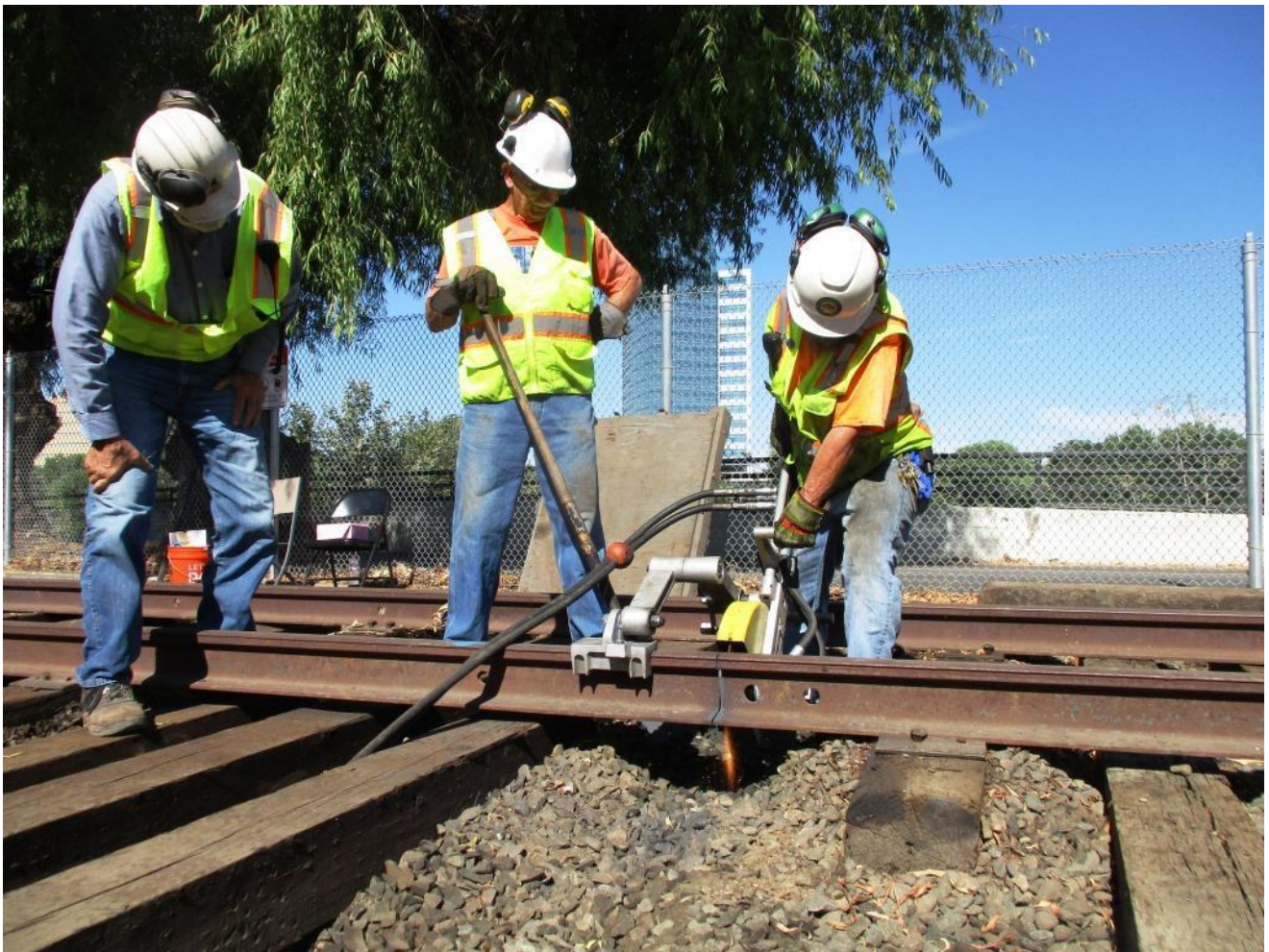
Alan watches as Clem and Joe finish the cuts necessary for replacing this segment of rail with the frog
