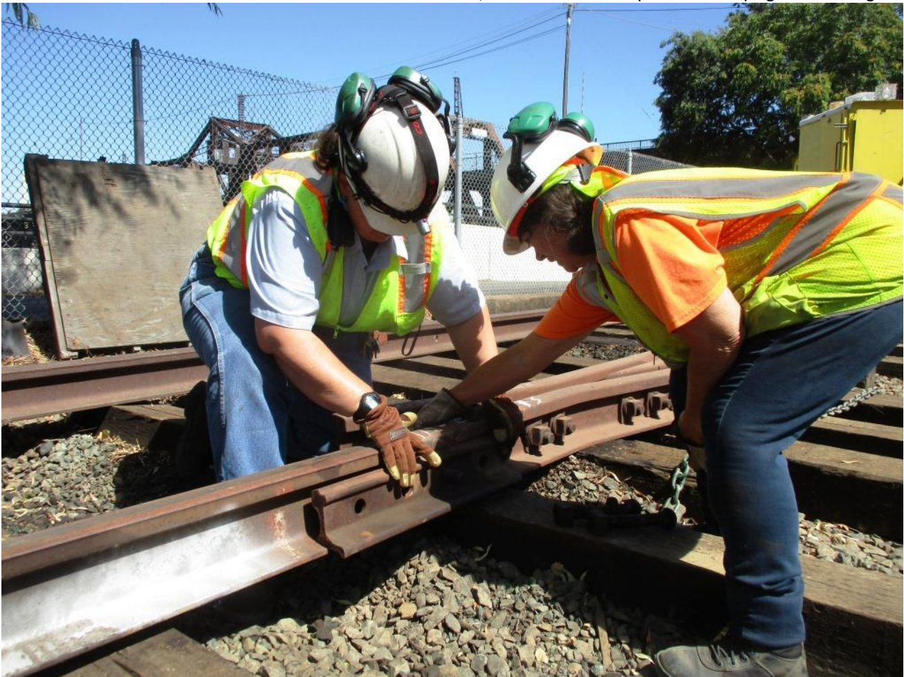
Heather and Pam attach joint-bars to connect the rail and frog together
