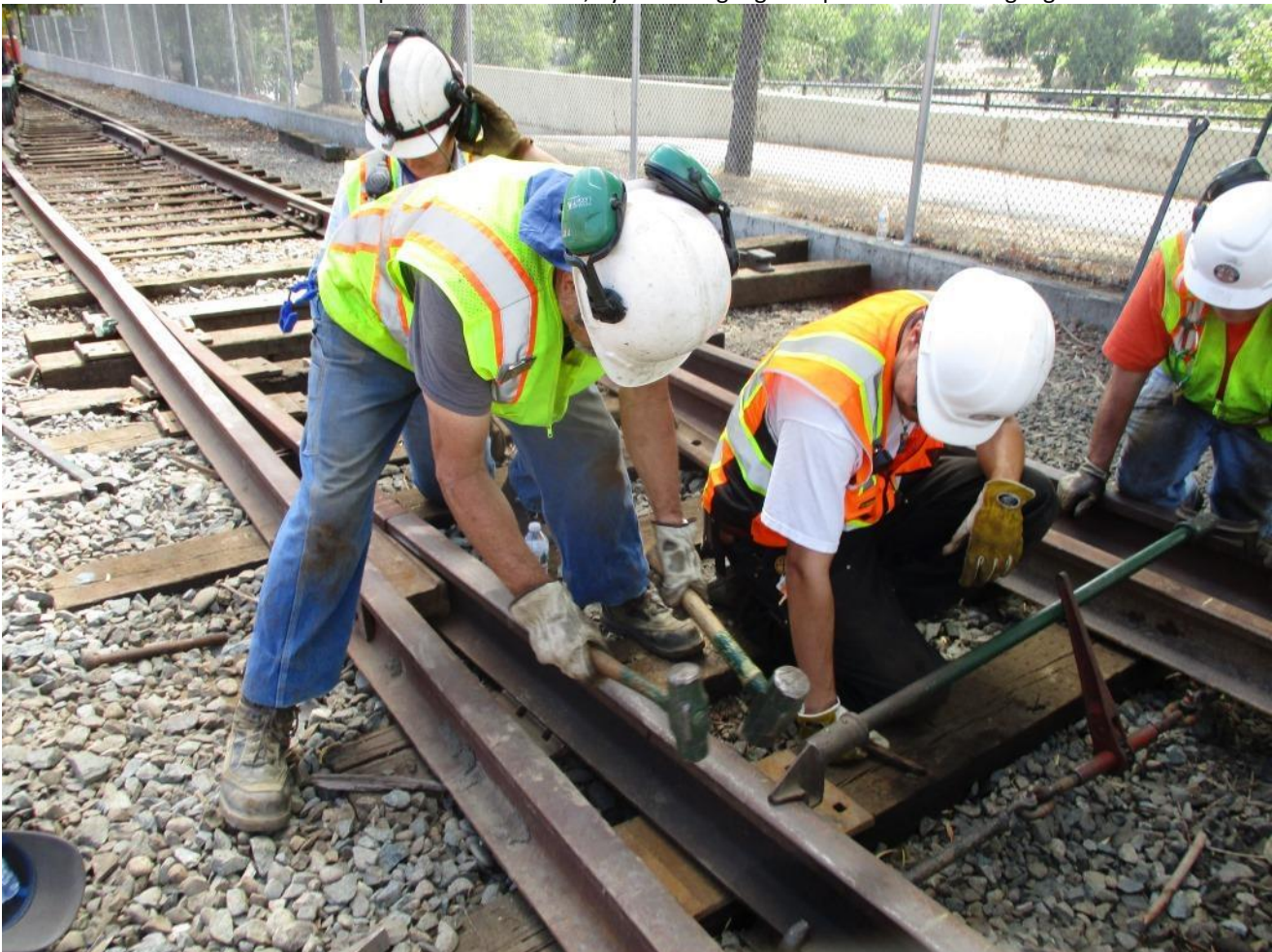
Ed demonstrates his patented "two-fisted hammering" technique for pounding tie-plates into place
