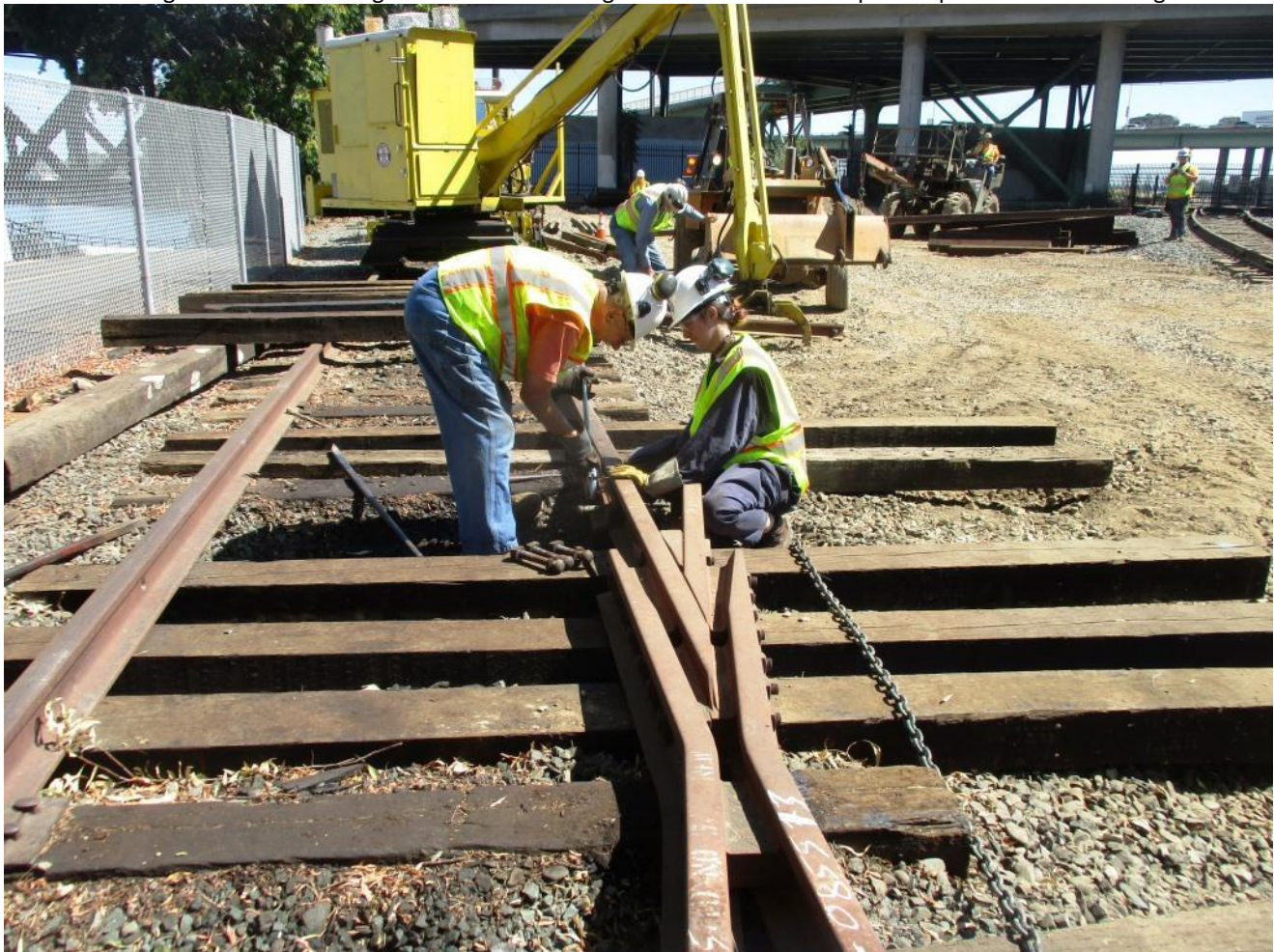
Clem and Samantha begin bolting the frog in place
