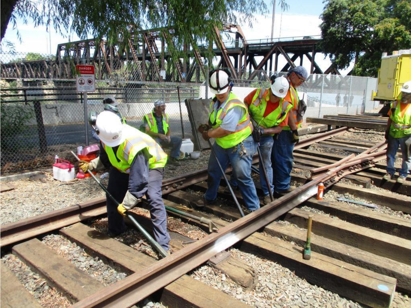
With the frog bolted in, Samantha, Heather, and Bill do a little "Gandy-dancing" to shove the rail into gauge
