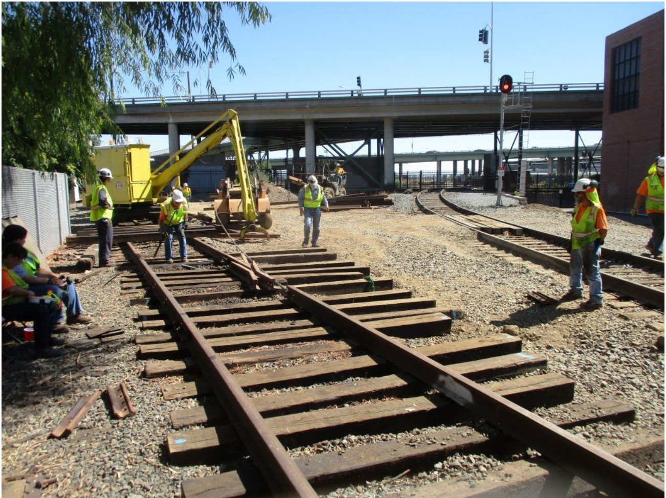
With a chain attached between the bucket and a stick of rail, Ed on the back-hoe pulls the rail up against the frog
