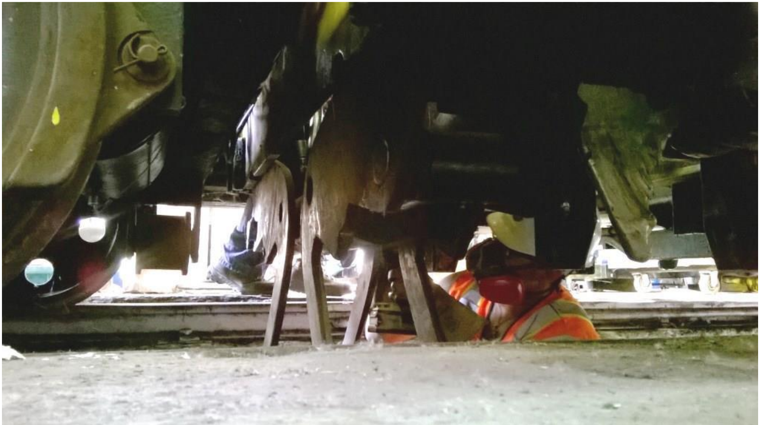
Kyle in the "pit of despair" working on the tie-shear's kickers
