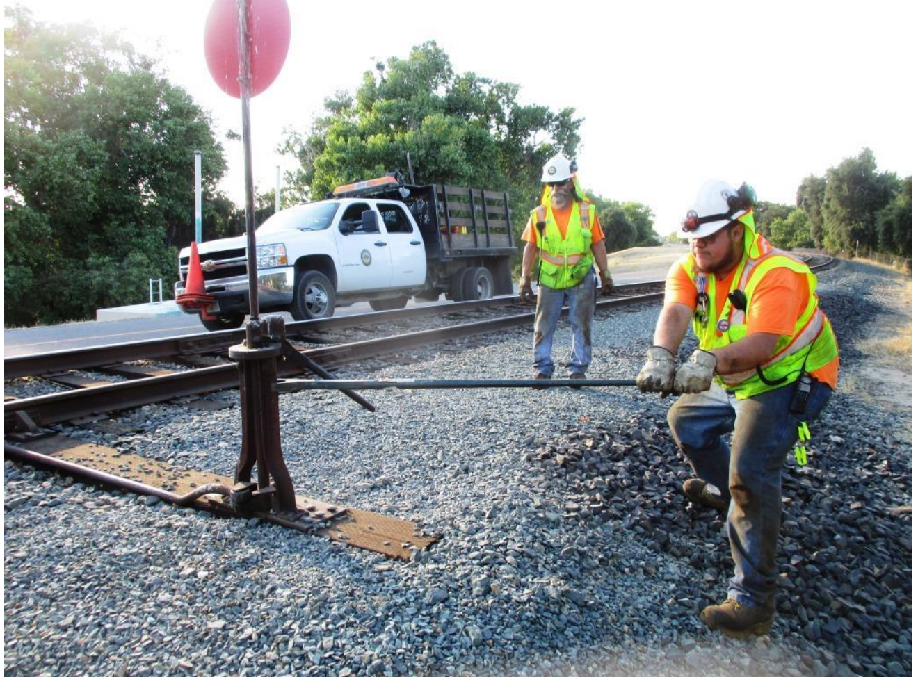
Chris makes subtle adjustments to the switch-stand
