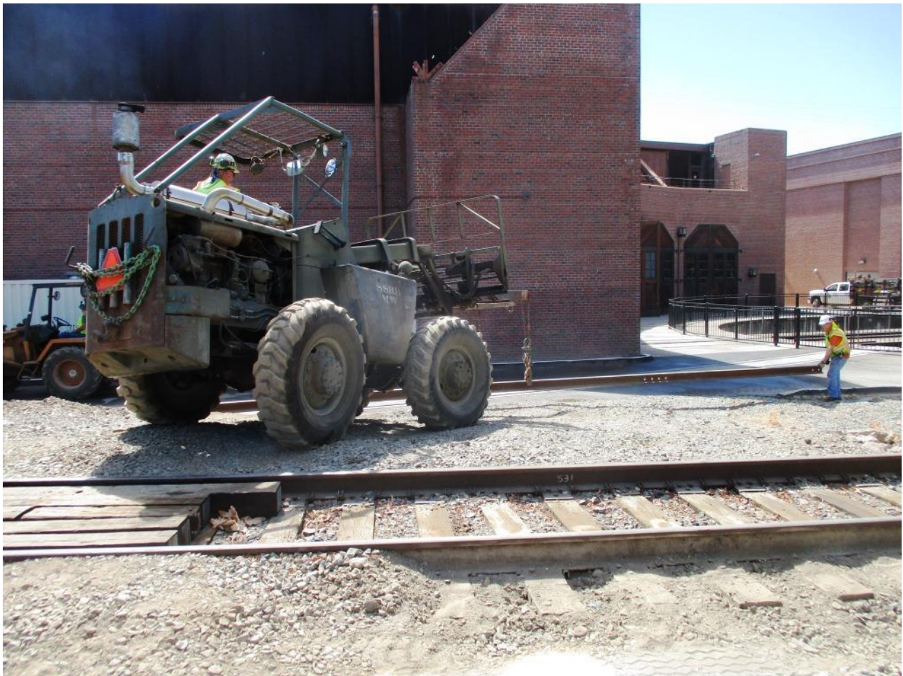
Bill guides the diverging stock-rail hanging from the forks of Big Green as Mike F. takes it down the hill to turn around
