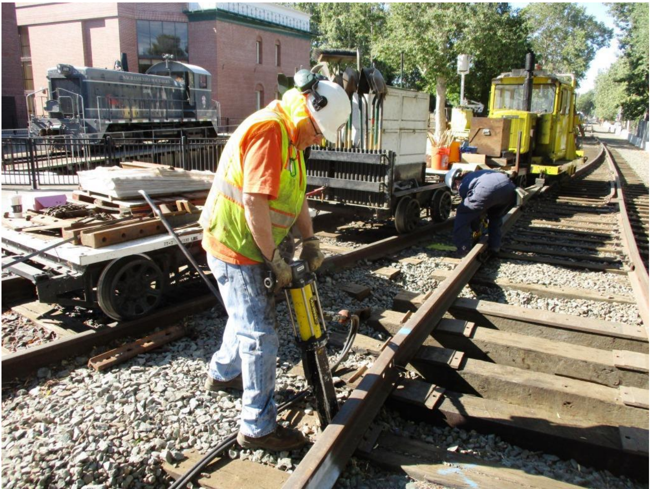
Bill uses the hydraulic spike-puller to pull spikes on the rail that will be replaced with the diverging stock-rail
