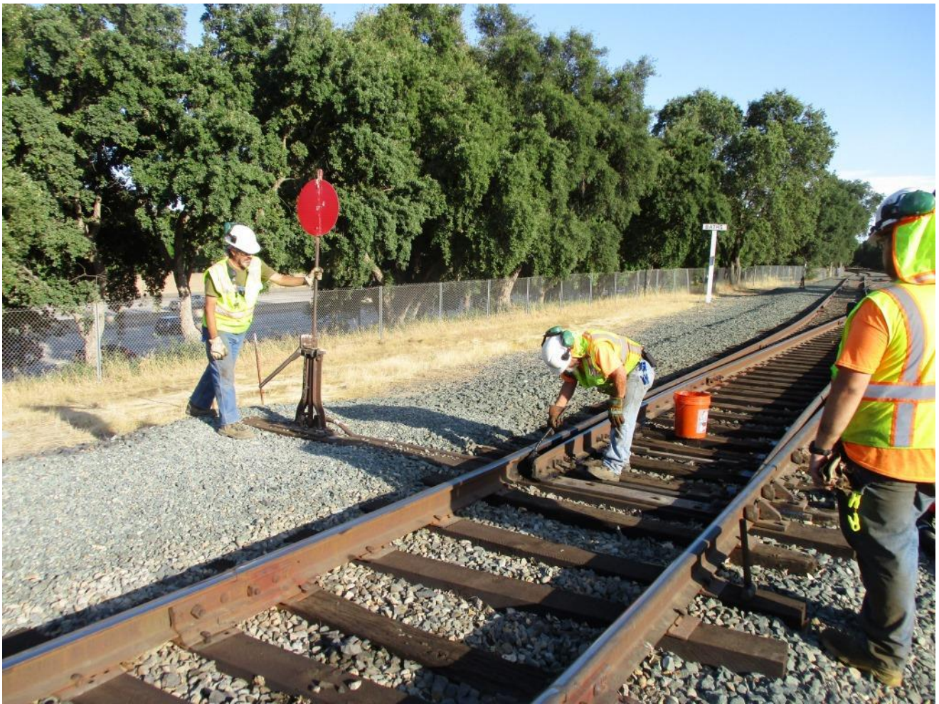
Ed exercises the switch machine as Joe slathers switch-grease on the components
