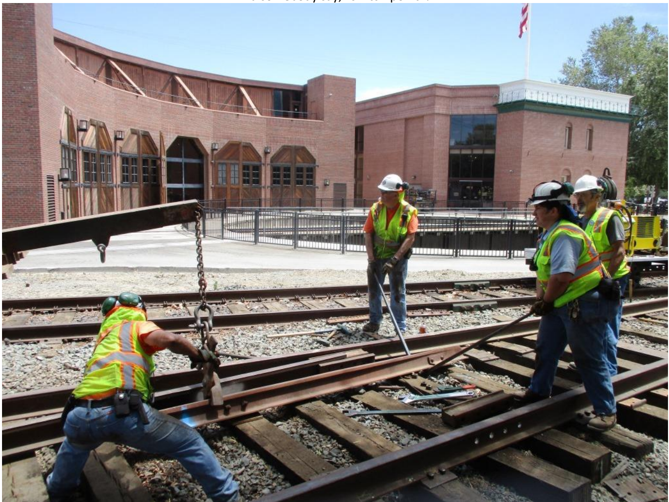
With the switch-point hanging from the stinger of Big Green, Joe, Bill, Ed, and Heather manipulate it into place against the heel-block
