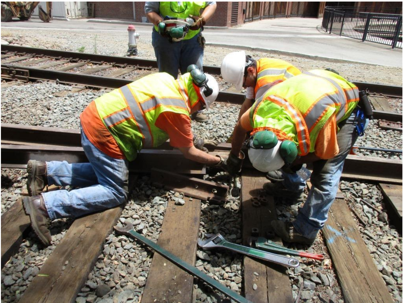
Bill, Kyle, and Joe shimmy around the weighty block to get everything lined up before the switch point can be installed
