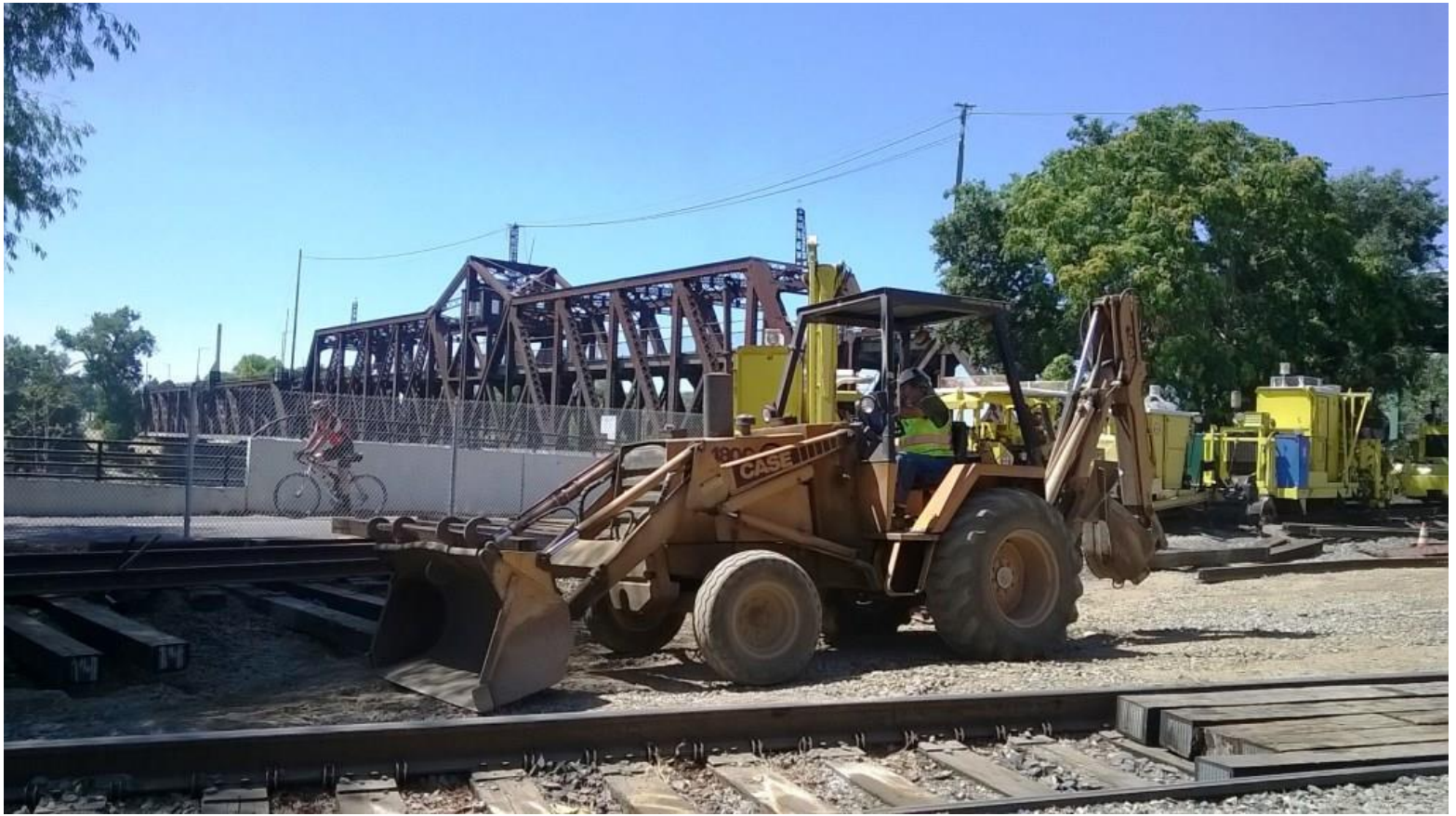
Ed uses the back-hoe to grade the roadbed for the diverging track being built behind the Museum
