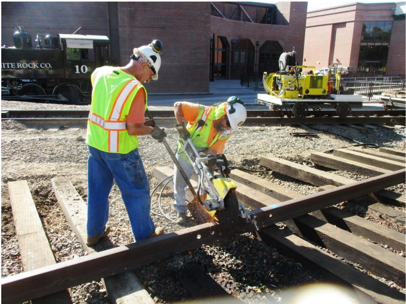
Clem uses a shovel to shield sparks from the rail-saw from bouncing back on Joe
