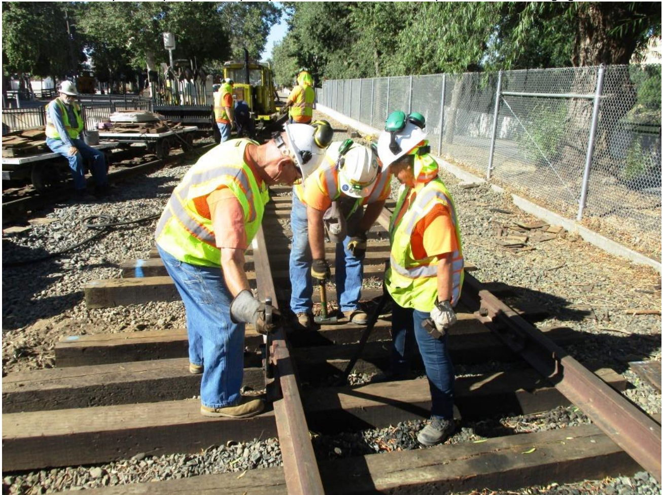
Clem, Mike F., and Pam take apart the north joint on the rail being replaced by the diverging stock-rail
